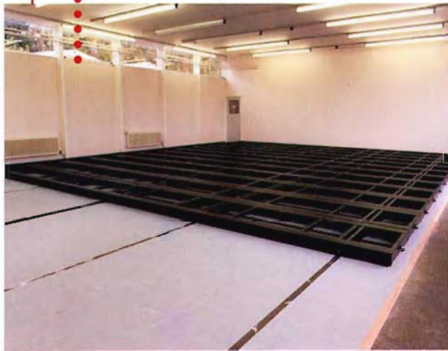
4 Mobile bases are mounted onto the tracks
