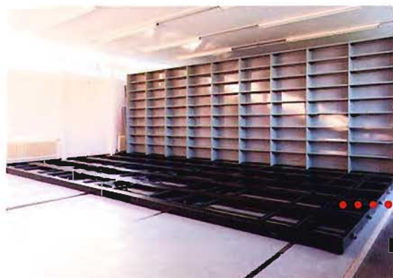
6 Shelving completed and awaiting end panels and drive wheels
